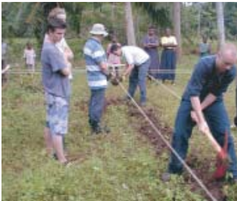
Digging the foundations of the Nutrition Centre
